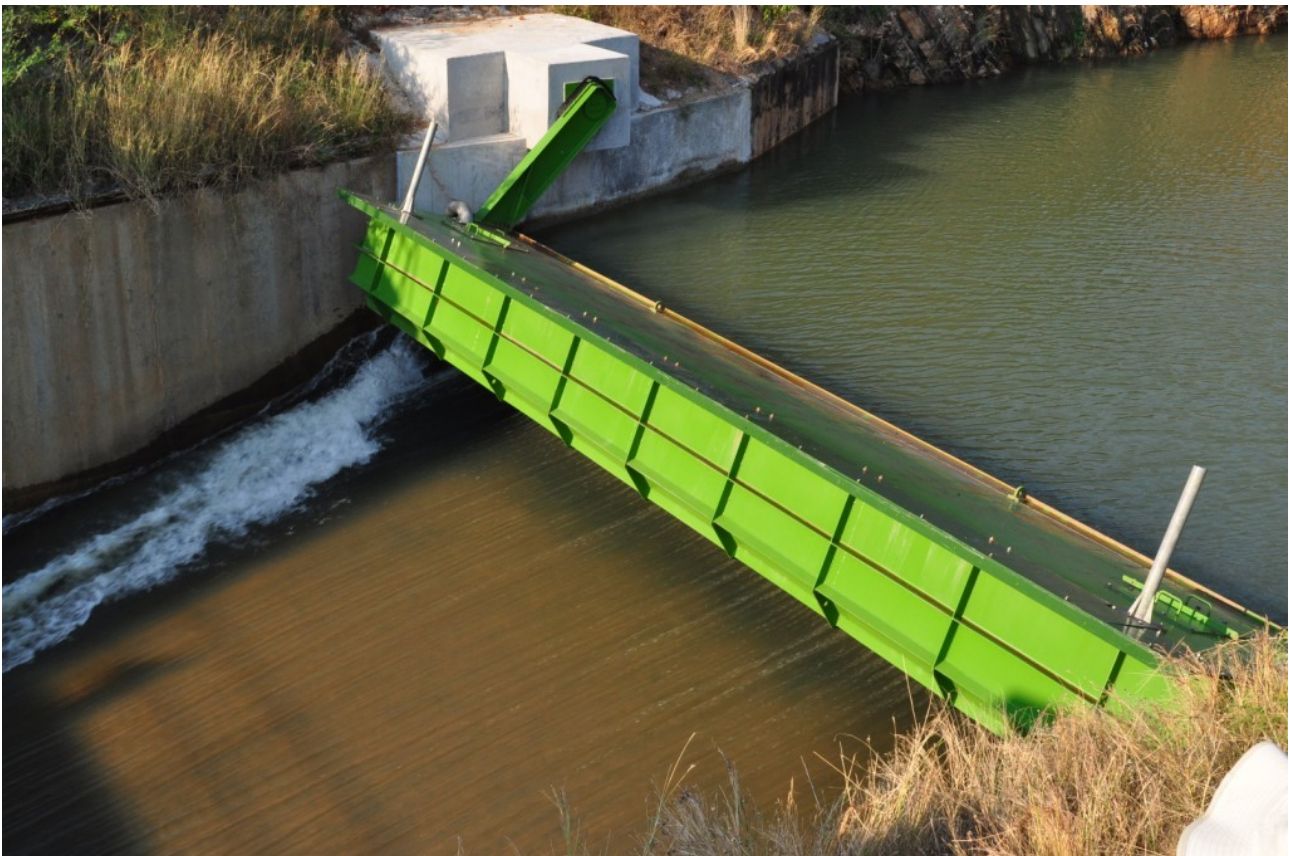
This photo shows a 12-m-wide by 1.5-m-high TOPS gate on the Mnjoli Dam in Swaziland. The gate is activated by a siphon and has opened automatically a few times already.
