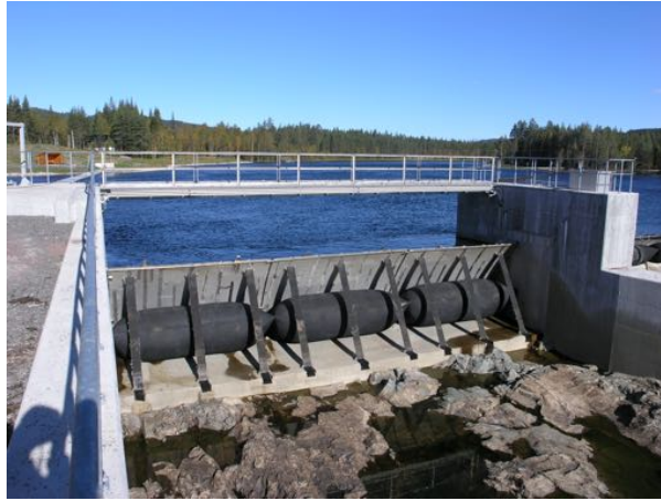
Figure 3. Flap gate with air bags (Obermeyer)
