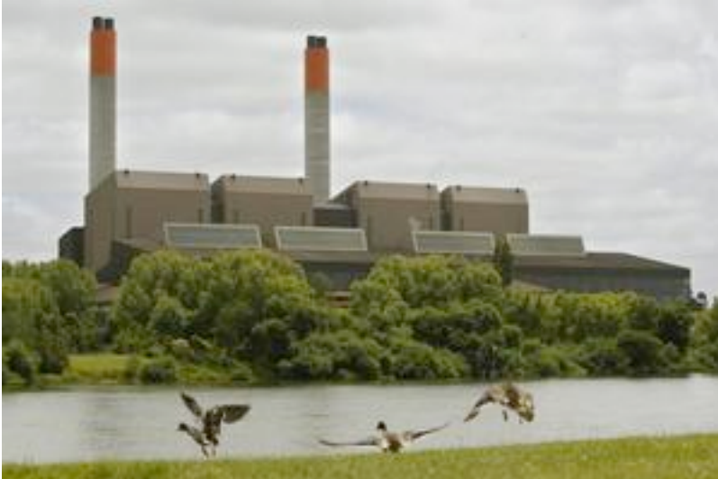
Huntly power station has used coal to generate power during dry periods. Photo / Amos Chapple
