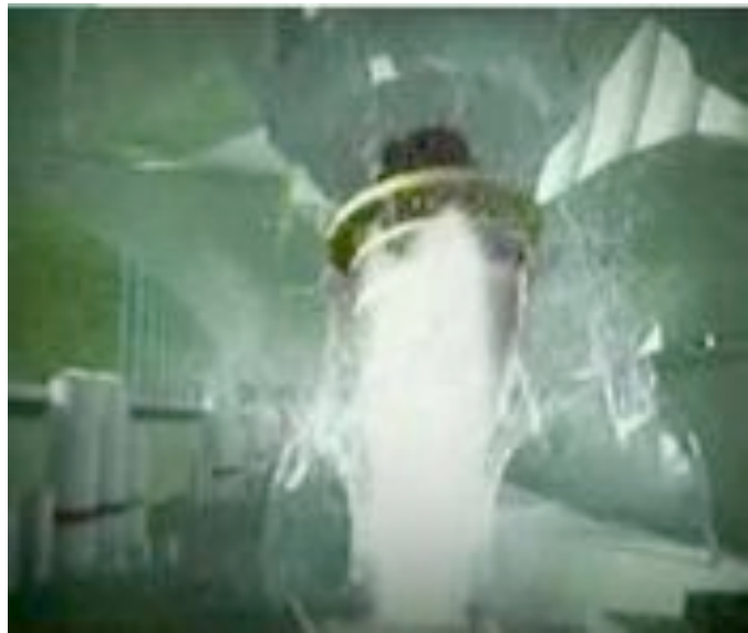
Figure 3 Unit 2 Generator rotor and turbine spinning above the generator floor level
