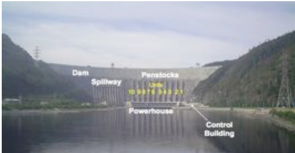
Figure 1 Dam and 6400 MW power station
